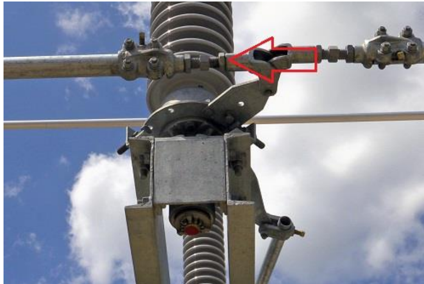
View of Turnbuckle Jam Nuts
