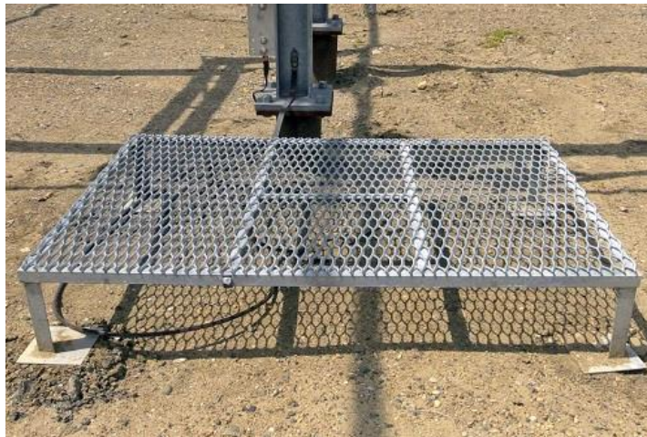
View of Grounding Mat
