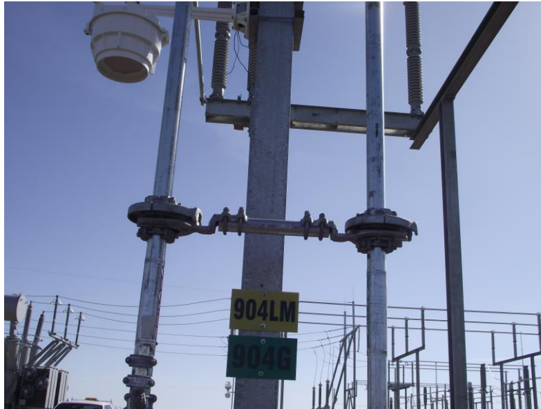
View of Switch Designation Sign
