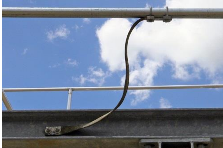
View of Main Drive Pipe Ground
