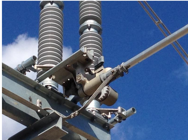
View of Ground Blade Grounding
