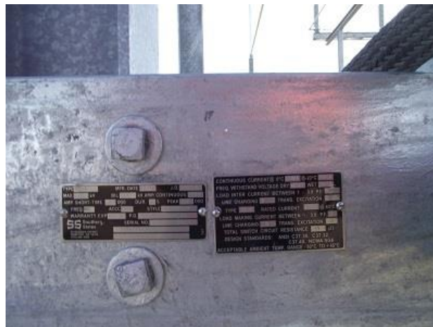
View of the Switch Name Plates
