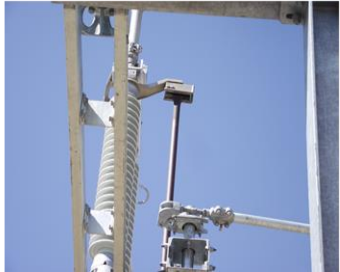
Examples of Proper Ground Blade Penetration
