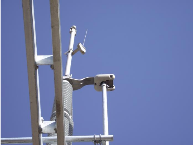
Examples of Proper Ground Blade Penetration
