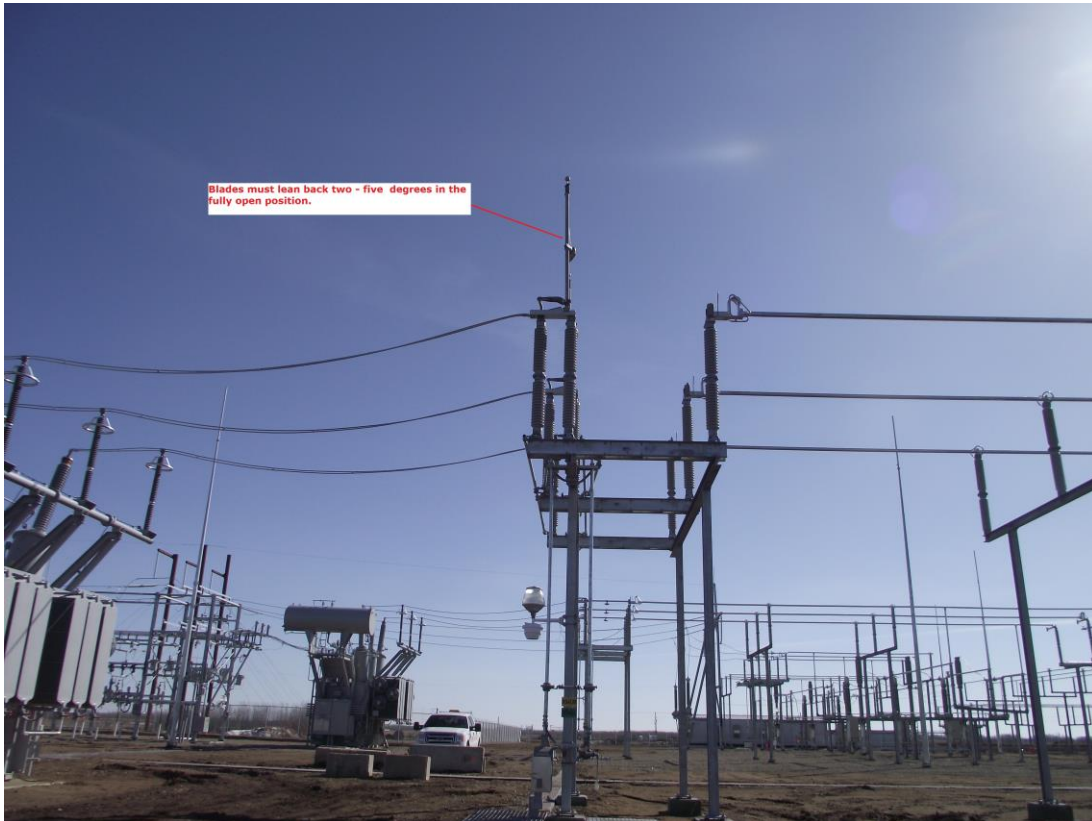
End Break Switch in Fully Open Position
