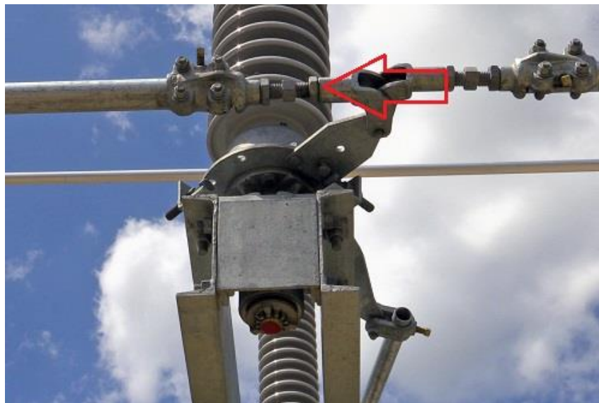
View of Turnbuckle Jam
