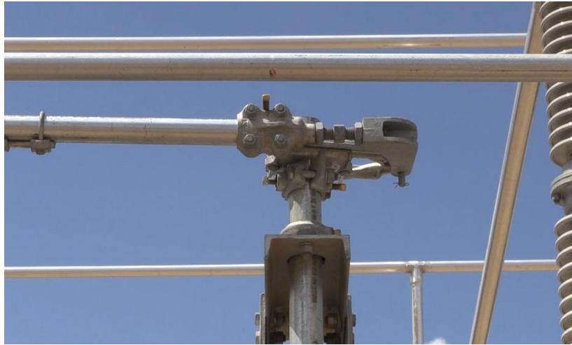
View of the Outboard (Fifth) Bearing where Toggle will be Present
