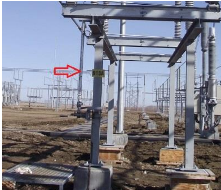
View of Switching Station Designation Sign
