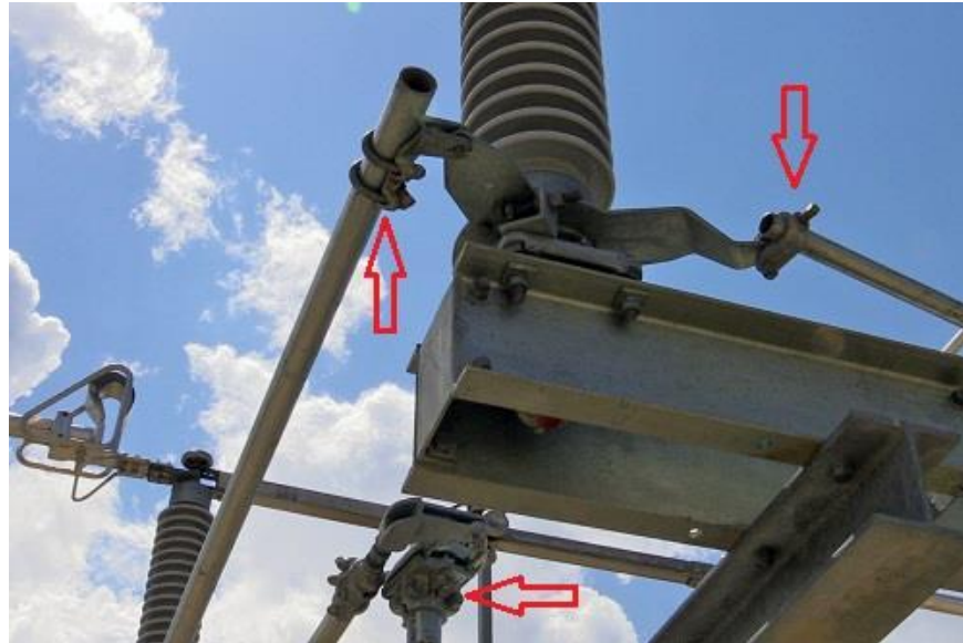
View of some of the Piercing Screws
