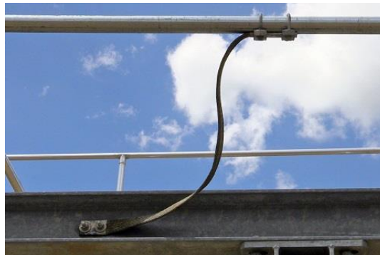
View of Main Drive Pipe Ground
