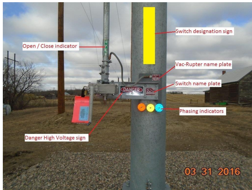
View of a Line Switch Designation Sign and other required signage
