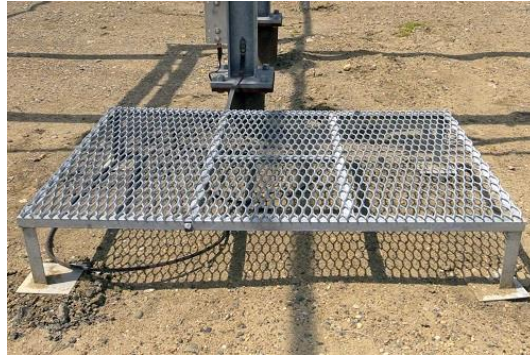
View of Grounding Mat
