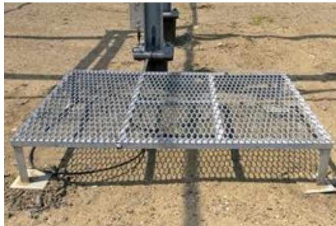
View of Ground Mat
