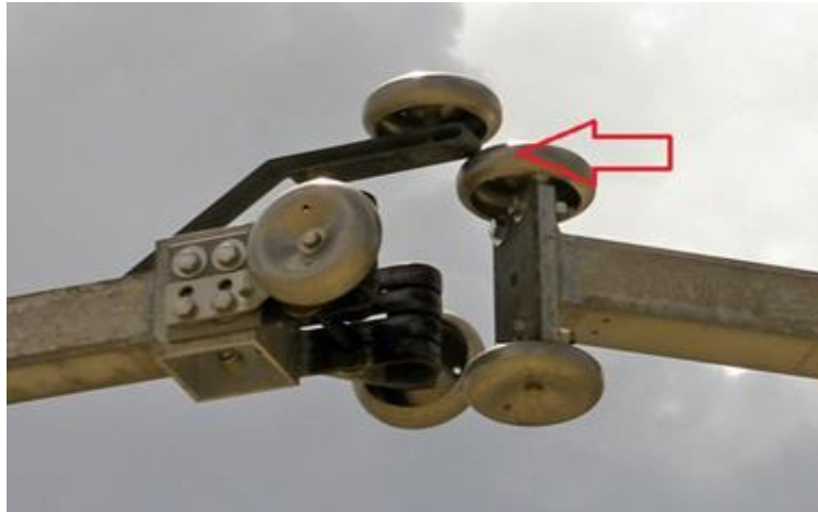
View of Arching Horns Making Initial Contact
