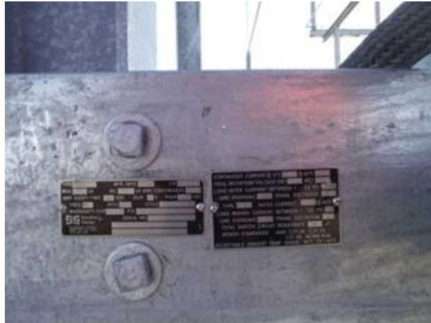
View of the Switch Name Plates
