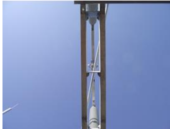
View From Under the Switch Blade Using the I-beam to Confirm Blade Alignment
