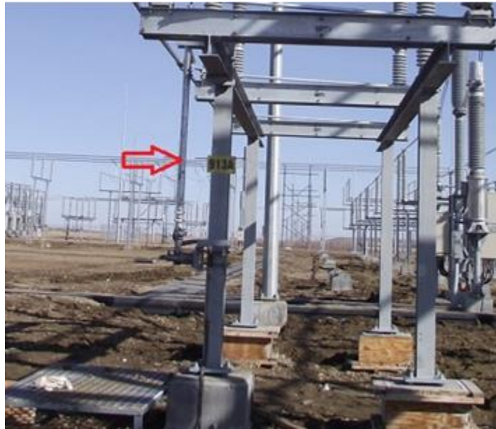
View of Switch Designation Sign
