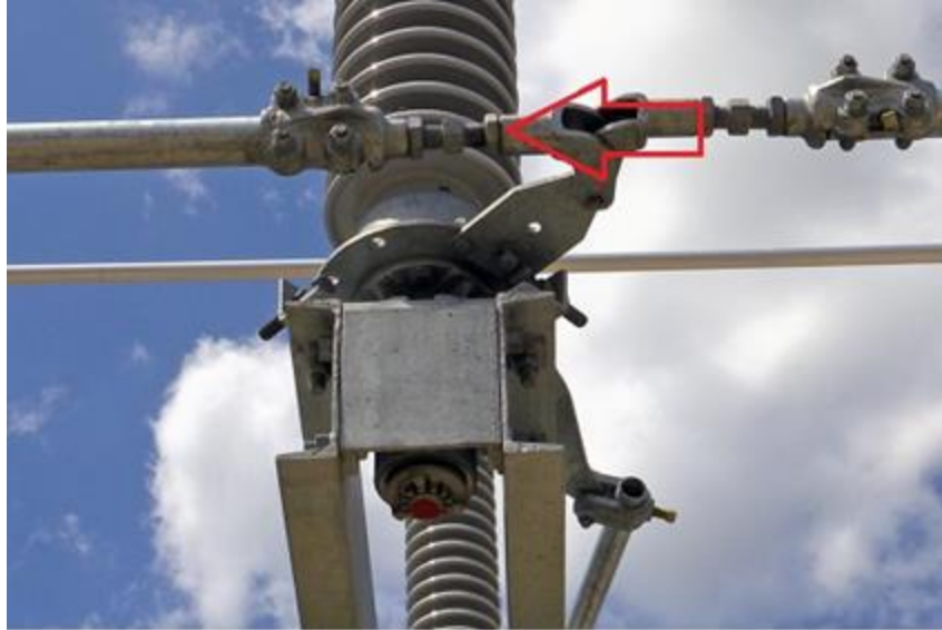
View of Turnbuckle Jam Nuts
