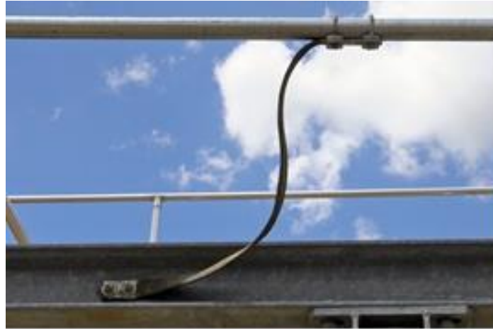
View of Main Drive Pipe Ground
