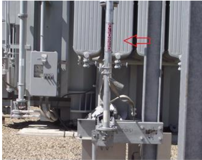
View of Closed Indicator Sign, Open is on Opposite Side of Pipe
