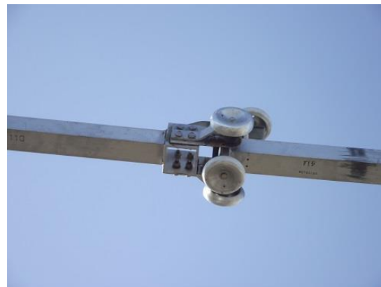
View of Contacts Making Proper Penetration in Fully Closed Position
